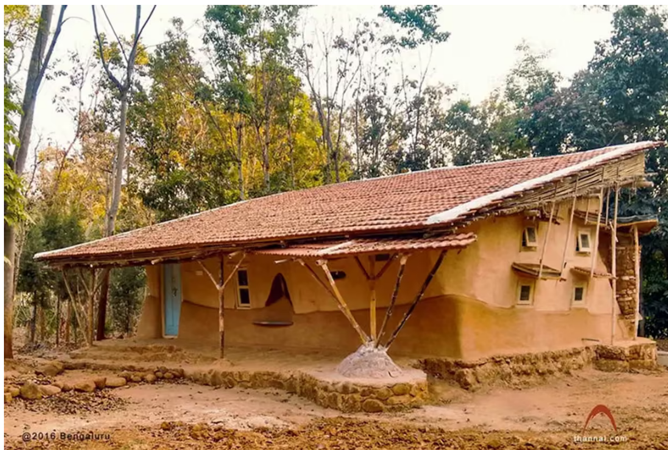
A wattle-and-daub cottage designed by Indian architects Thannal, who specialise in natural building techniques. Photograph: Thannal
